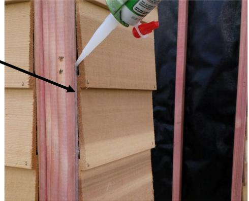
Step 11: Nail 15 x 17mm beads on front corners and beside doorway as shown, using 4 x 50mm stainless steel beading nails, per bead. Ensure top is flush with top plate.
