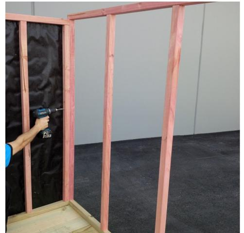
Step 8: Select remaining panels, predrill and screw together as shown.
