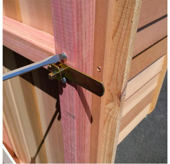
Step 29: Attach Cedar door blocks to both front wall panels, hard underneath roof.
