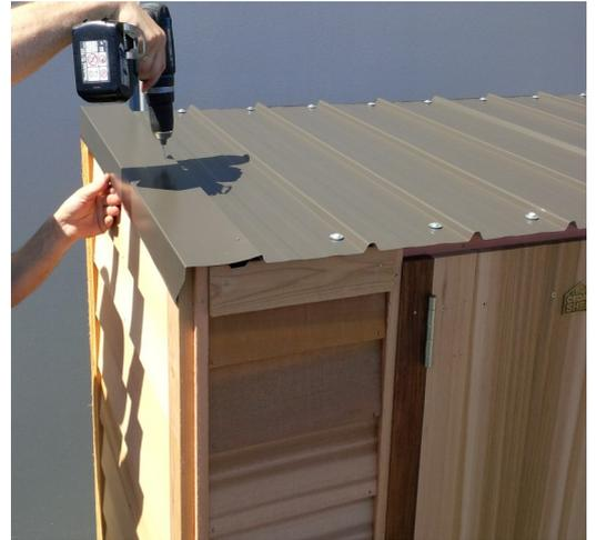
Step 31: Using 3 rivets, rivet ends of spouting to barges and rivet 1 rivet into roof sheet.
