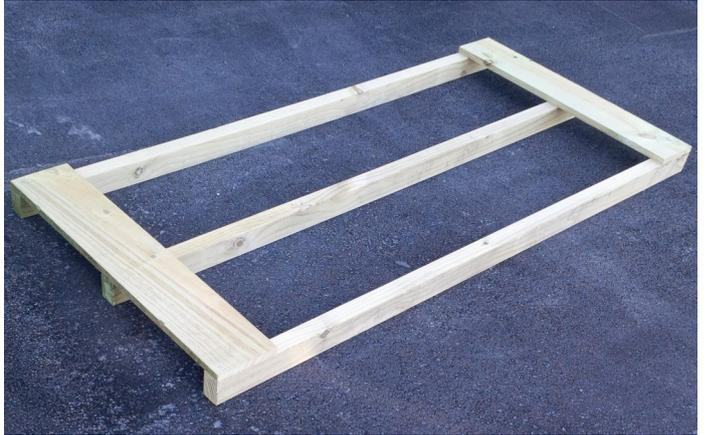
Step 2: Lay out remaining floor boards. Measure diagonals to ensure measurements are equal (i.e. floor is square). Rip down last floor board to suit gap, and nail off floor with 50mm flooring nails (2 nails per Joist, per board).
