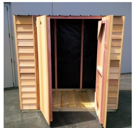
Step 25: Using 40mm screws, screw padbolt as shown, to the edge of the Left hand door ensuring padbolt will protrude at least 10mm into the floor when in locked position.
