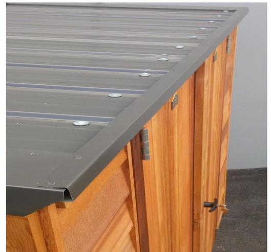
Step 32: Rivet ridge flashing to barges and roof sheets as above.
