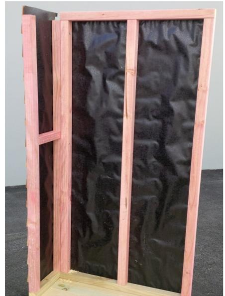
Step 5: Using a 6.5mm drill bit, predrill stud then screw wall panels together using 75mm tek screws (3 per join), ensuring end wall panels are inside side wall panels as per wall plan.
