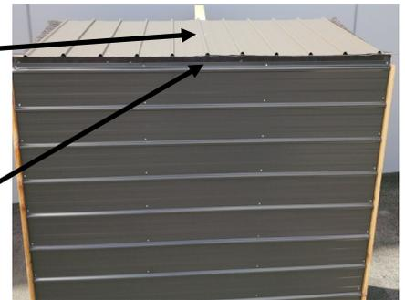
Step 21: Screw the first sheet with a 50mm roofing screw with washer. Screw through the rib of sheet into back wall top plate.
