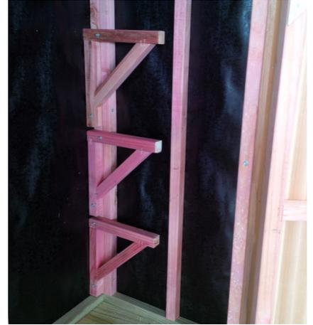
Step 33: Screw plywood shelves to brackets with 40mm screws, (6 per shelf).
