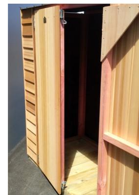
Step 27: Fasten Top padbolt as per above steps. Drill 10mm hole into underside of top plate.
