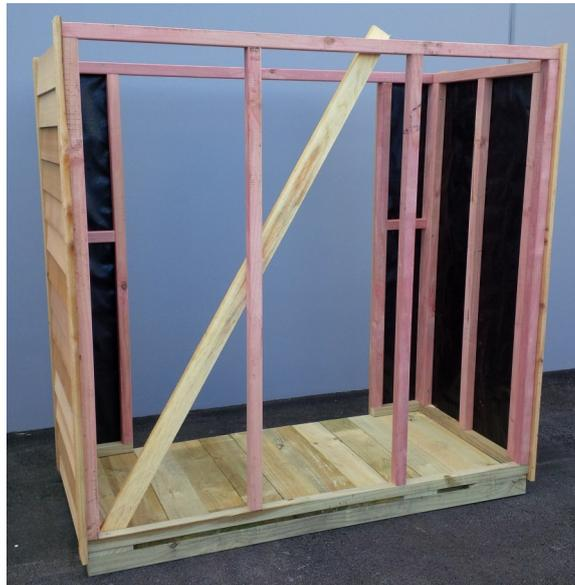
Step 15: Using 30mm clouts, nail building paper vertically to outside of framing, starting at one edge, leaving a 25mm overhang at the bottom. Trim edge of paper flush with top plate and edge of studs as shown. Repeat above to complete back wall.
