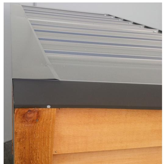
Step 31: Touch up all nail heads and rivets using colour steel paint supplied.
