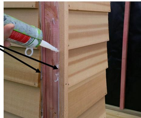
Step 13: Nail corner clashing's onto corners as shown, using 4 x 50mm stainless steel beading nails, per bead. Ensure top is flush with back and top plates.
